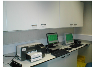
FMS work station
